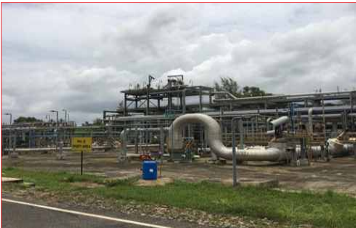
Shaft Area of Padur
