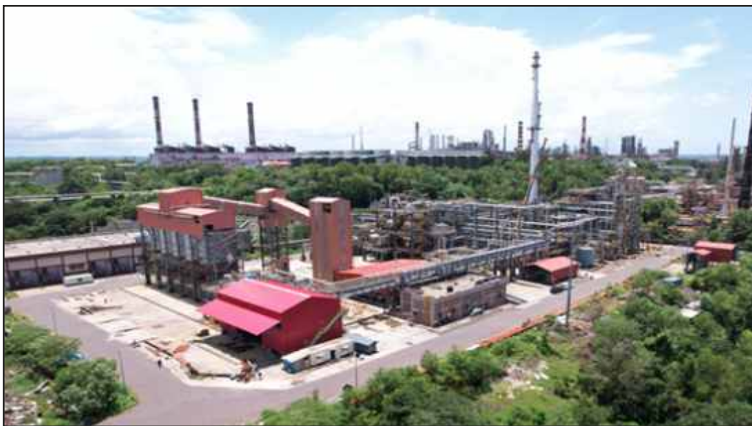
Sulphur Recovery Unit (SRU), Mangalore
