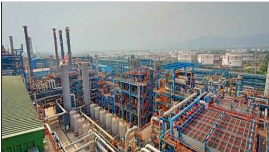
Hydrogen Generation Unit, Visakh Refinery
