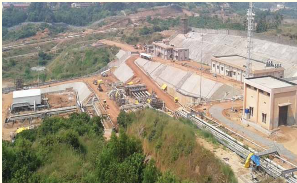
Overview of Mangalore Site
